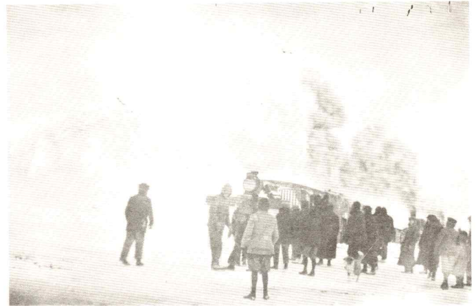
A snow plow clearing the RR tracks in the 1920's
